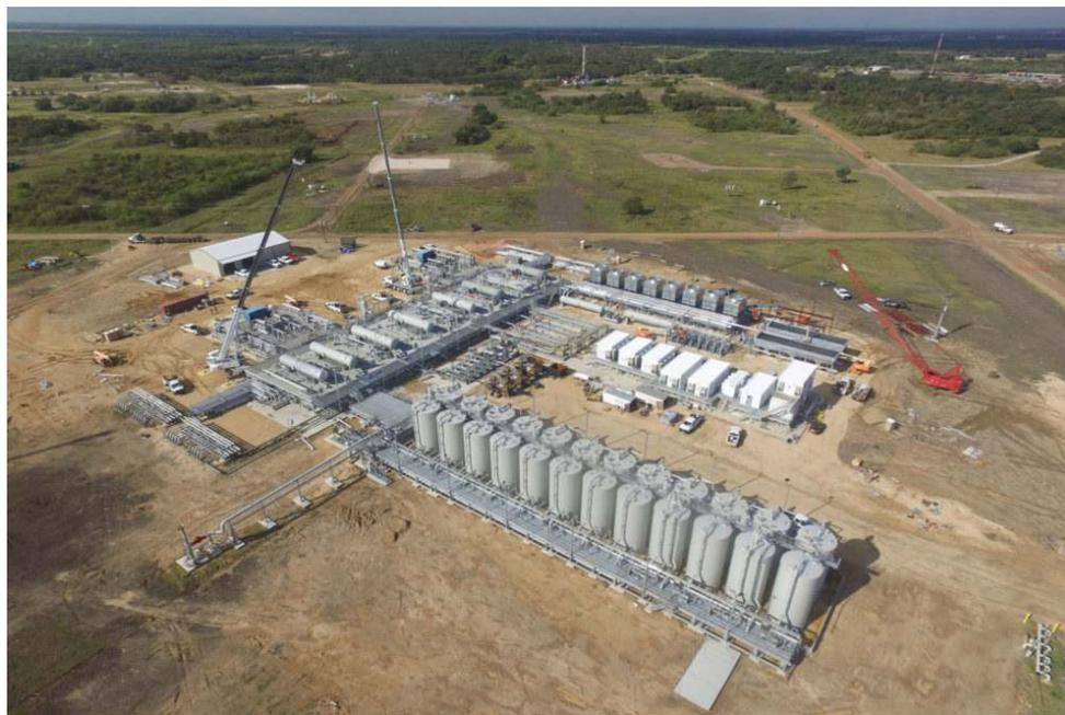
CO2 emissions captured by the Petra Nova power plant are piped 80 miles to the West Ranch oil field and used to recover hard-to-reach oil. COURTESY OF NRG
